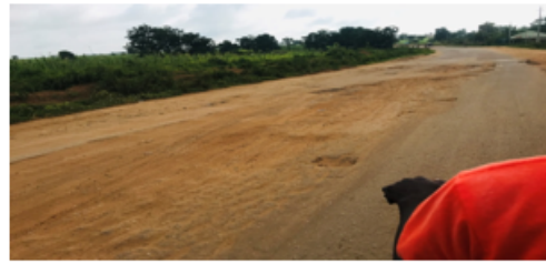
Fig 3: Some Distresses (Raveling) Located at about 1.1 km from the Origin
