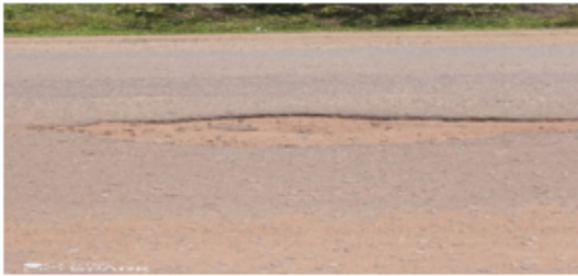
Fig 2: Some Distresses Located at about 7km from the Origin (Low-cost Junction)
