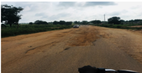
Fig 3: Some Distresses (Raveling) Located at about 1.1 km from the Origin
